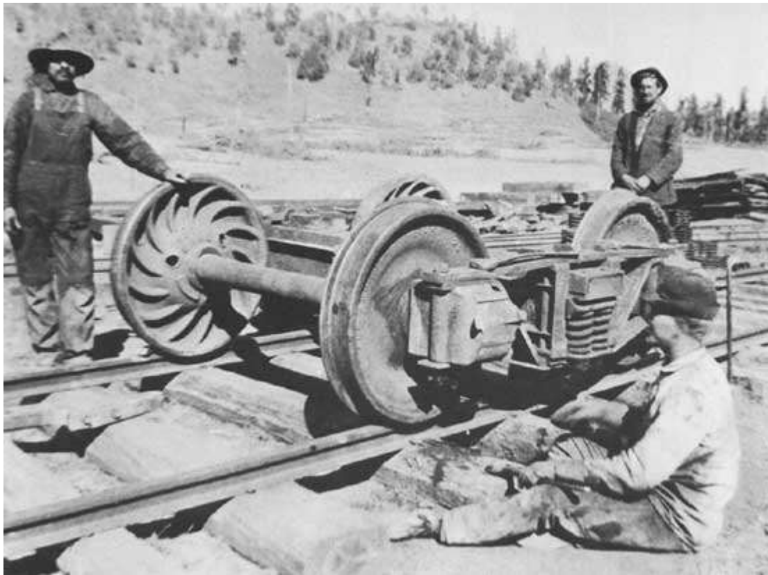
Figure 61. Tree "car tanks"—railway mechanics—working on an arch-bar freight car truck at Kettner, circa 1908. This type of truck, bolted together of individual parts, was soon superseded by massive cast trucks. ( John Bigley collection )
