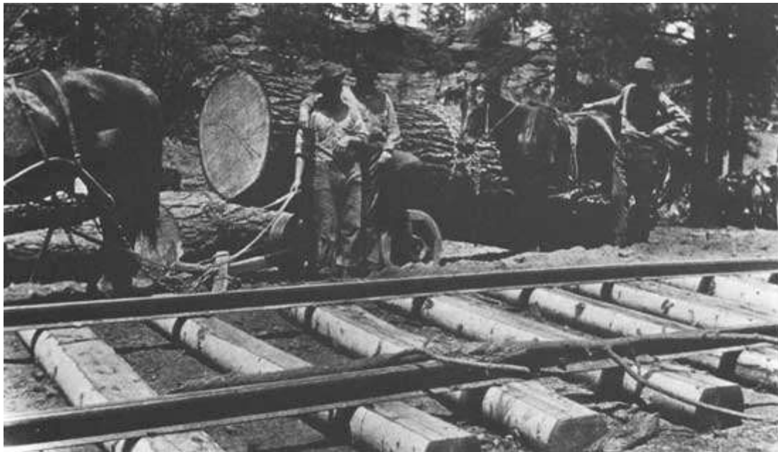
Figure 21. Some interesting details of logging practices are evident in this view. The large log was being skidded on a low-wheeled truck called a "bummer." Its small wheels required flat and relatively firm ground for its use (Bryant 1923:185). The railroad spur was laid with aspen ties, an unusual timber for the purpose. Note the spikes driven close to the sides of the ties, indicating an intention to use the ties at least once more on another spur line. The spikes were driven on the opposite sides for the second use. ( Cibola National Forest collection )
