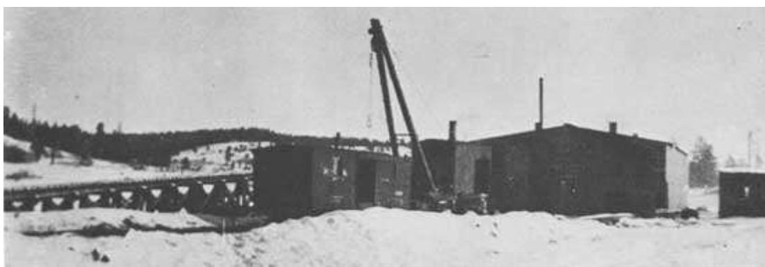
Figure 62. Winter view of the Sawyer roundhouse, circa 1908-1913. One of the American Lumber Company log loaders was spotted nearby, probably for repairs and maintenance during the slow winter months. ( John Bigley collection )
