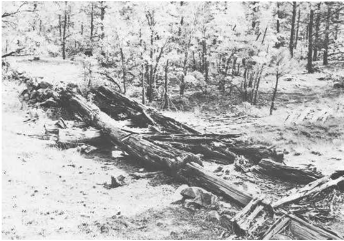
Figure 34. Three span cribwork trestle, 47.9 feet in length, on Pine Canyon railroad of George E. Breece Lumber Company, September 30, 1985. (By David "A" Gillio. USDA—Forest Service photograph)
