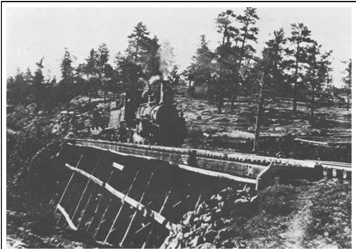
Figure 27. The ancient locomotive No. 4 of the Zuni Mountain Railway crossing a framed timber trestle. The location of this view is probably along the main line between Kettner and Thoreau in Cottonwood Canyon. ( Cibola Notional Forest collection )
