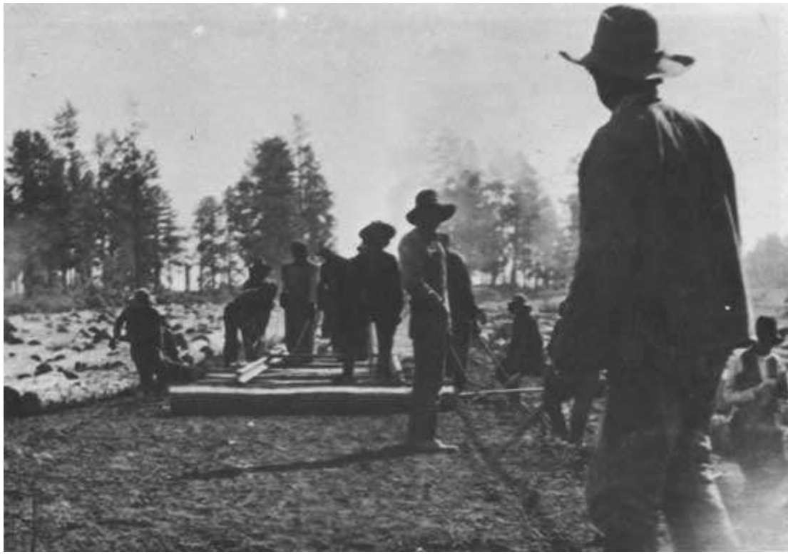
Figure 59. Laying track for the Zuni Mountain Railway on freshly graded roadbed. Logs had already been yarded to both sides of the new spur track ready for loading on the cars. ( Cibola National Forest collection )
