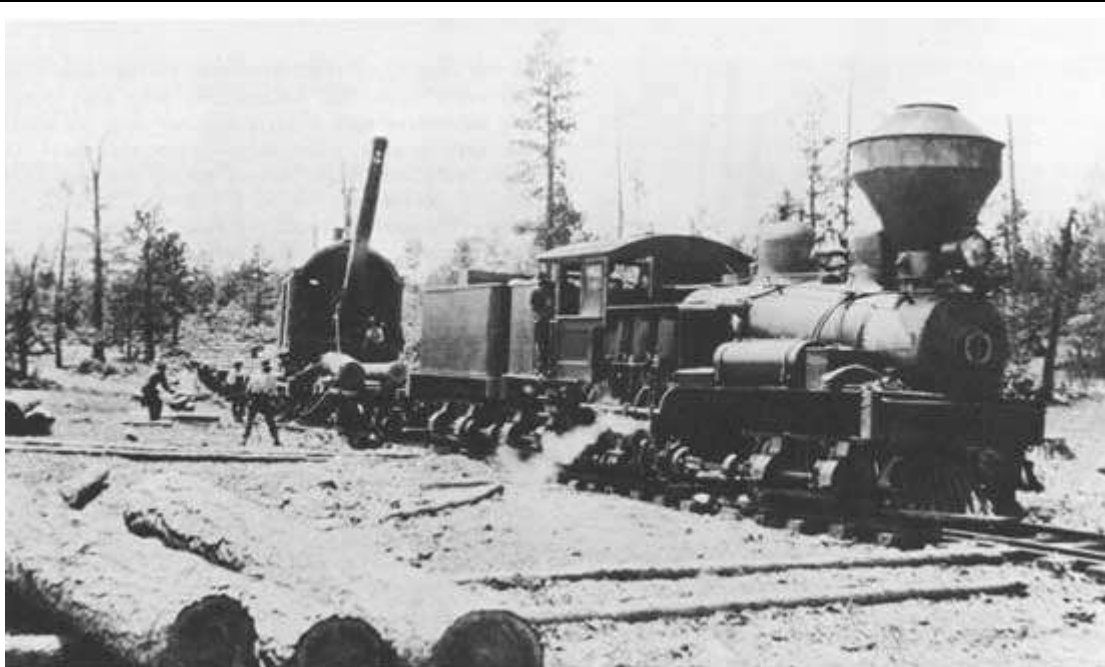
Figure 39. Loading logs on the McGaffey Contracting Company cutting. Shay locomotive Number 1 waited while the Barnhart loader hoisted the 16 to 20 foot pine logs onto the cars. After each car was loaded, the loader moved back one car length to repeat the process. The loader rode on car-top rails.
