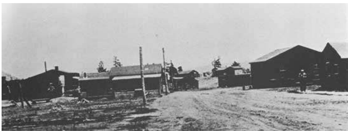
Figure 25. The main part of the logging camp at Sawyer on the American Lumber Company. On the extreme left can be seen part of the locomotive cooling trestle; next to it is the "roundhouse," used for minor repairs to the locomotives. On the track can be seen the Climax gear-drive locomotive. Zuni Mountain Railway No. 8. ( Cibola National Forest collection )
