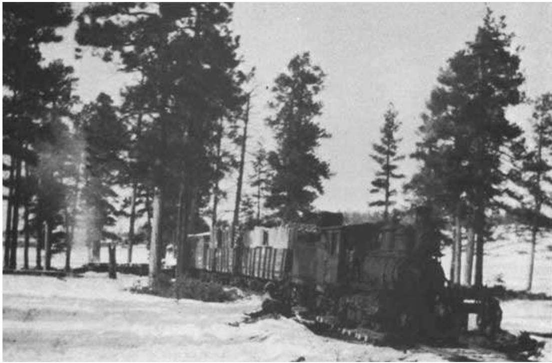
Figure 52. A borrowed Santa Fe Railway locomotive, Number 2303, off the rails on new logging track of the Zuni Mountain Railway, January 4, 1906. ( V. J. Glover collection )
