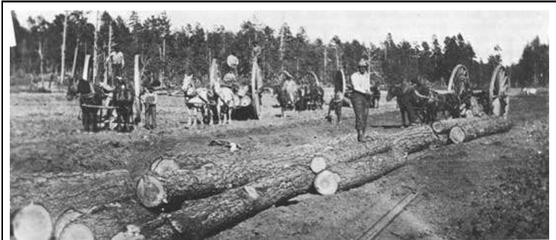
Figure 18. Skidding logs to the railroad with big wheels on the American Lumber Company. ( Cibola National Forest collection )
