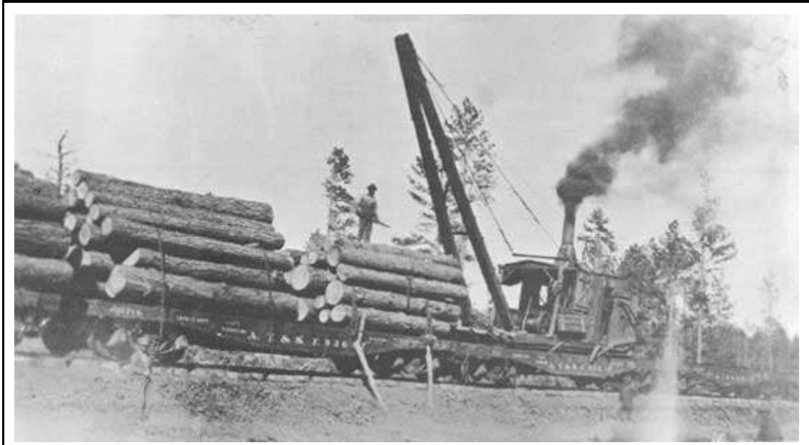
Figure 15. Loading standard 16-foot logs on Santa Fe Railway steel log cars. This steam loader is equipped with a rigid boom, and slides from car to car on steel skids. ( Cibola National Forest collection )
