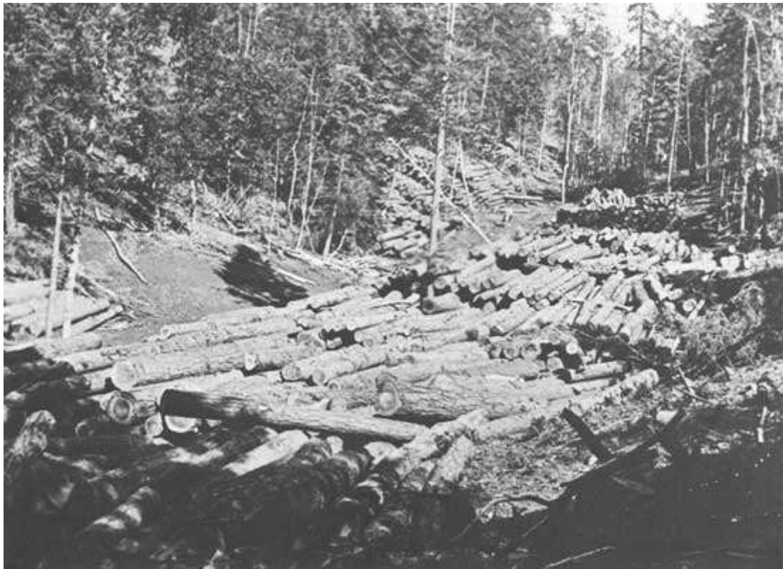
Figure 19. Log landing along a future spur track. American Lumber Company. These logs have been yarded in a little valley preparatory to loading on the cars when the spur track is built. It appears the roadbed has already been graded. ( Cibola Notional Forest collection )
