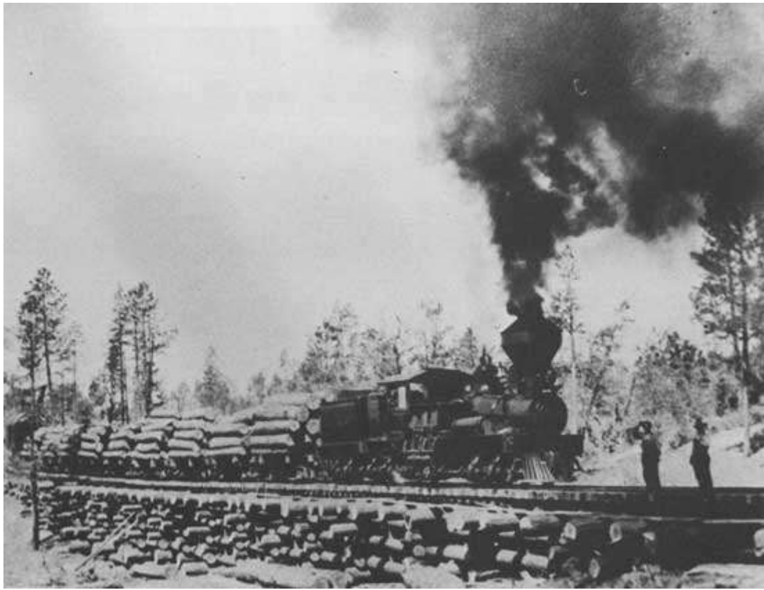
Figure 40. McGaffey Contracting Company log train heading for the mill. The Barnhart steam loader at the rear of the train rode on an empty log car from one loading point to another. The train was crossing a very large cribwork log trestle, sometimes called a "pig—pen" trestle. ( Robert Searle collection )
