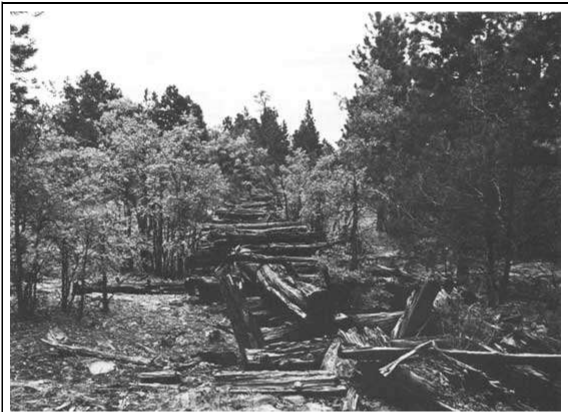
Figure 33. Curved cribwork trestle on Pine Canyon railroad of George E. Breece Lumber Company, September 30, 1985. This structure spanned 211.6 feet with 13 spans of logs; it was built circa 1924-1925. (By David 'A' Gillio, USDA—Forest Service photograph)
