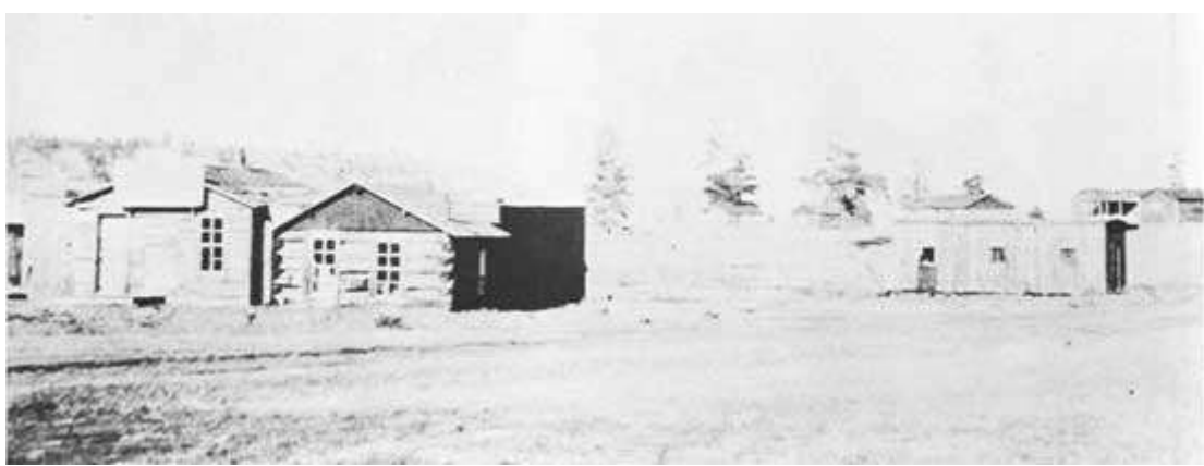
Figure 64. The logging camp at Sawyer on the American Lumber Company holdings. A wide variety of building construction was apparent, including some structures intended for haulage on railroad cars. (Cibola National Forest collection)
