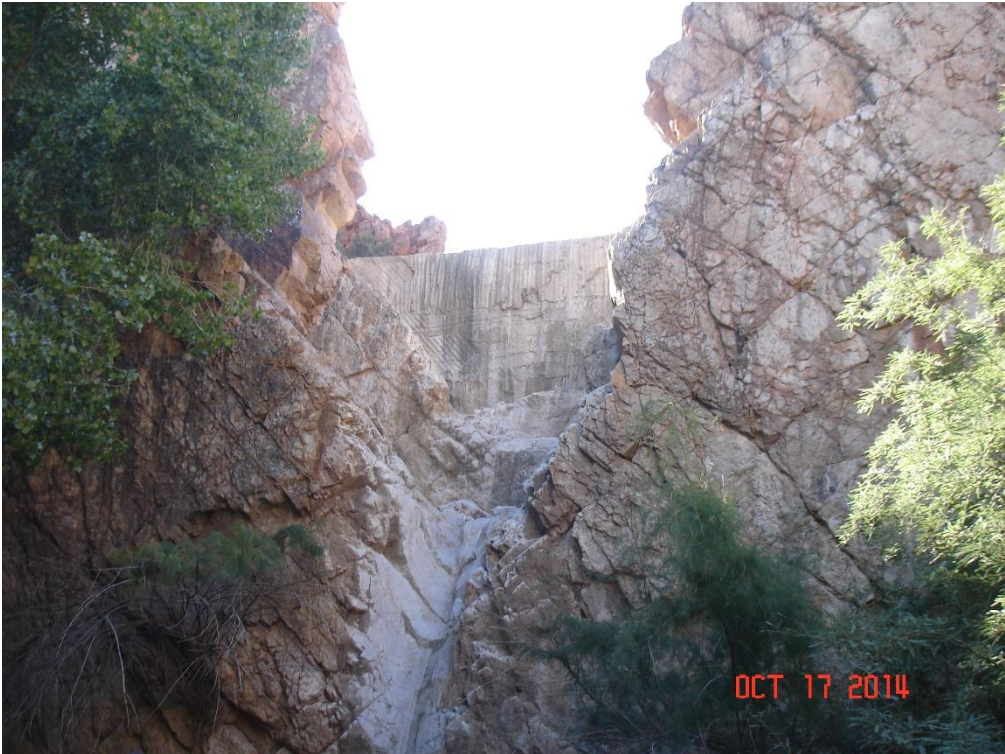
The dam from the downstream side
