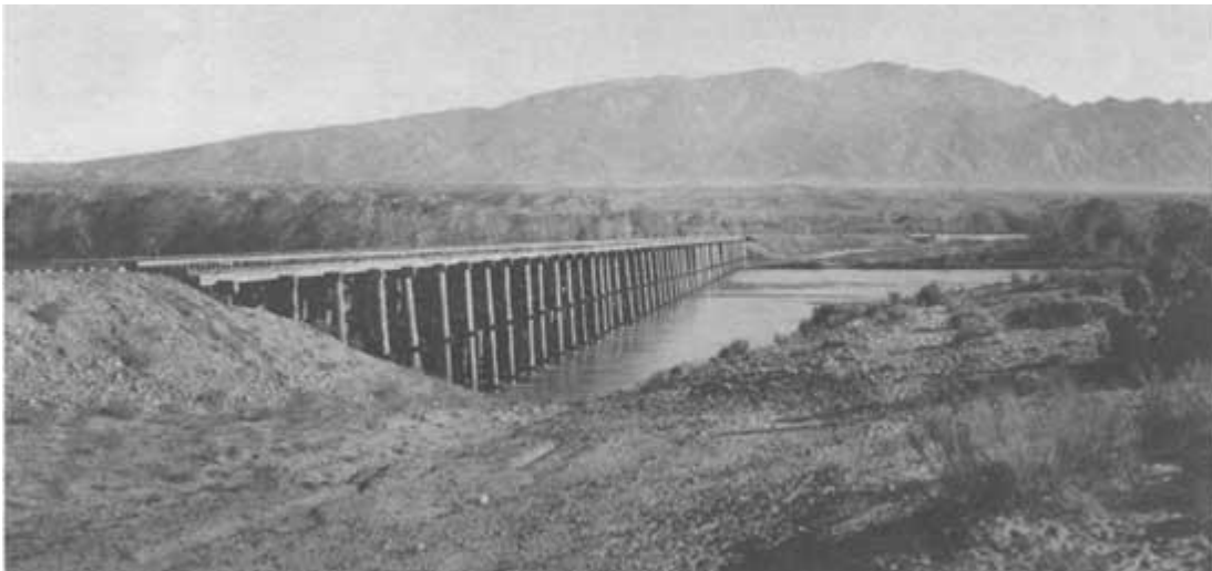
Figure 4. Rio Grande trestle soon after its construction in early 1923. Of standard AT&SF design, this structure was built of piles driven into the bed of the river. The embankment on the far side of the river shows the grade as the track begins its climb into the hills on the west side of the Rio Grande behind the camera. (Photo By M. E. Hanna. Albuquerque Public Library collection)
