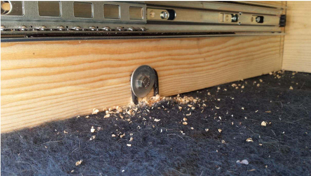
Heavy duty drawer sliders from Lowes, and fender washers through bolted on the rear tie downs.
