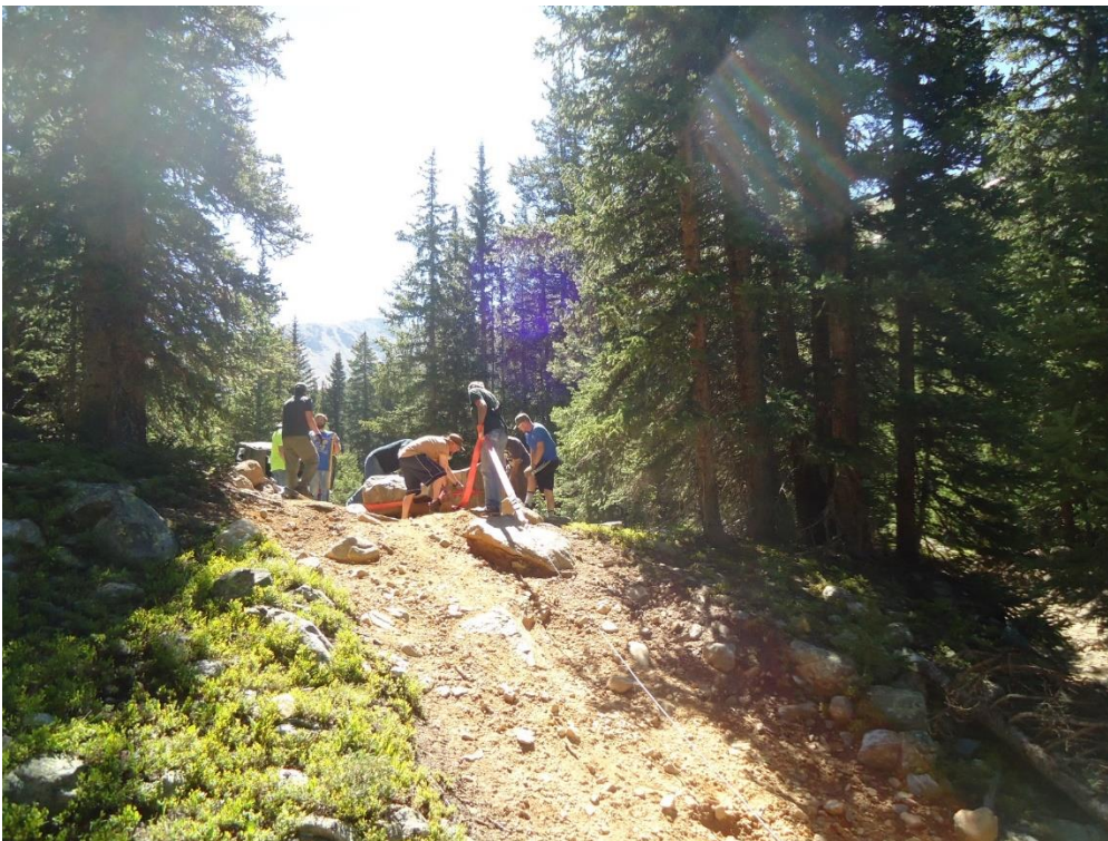
Blocking the illegal bypass to prevent further damage to the area.
