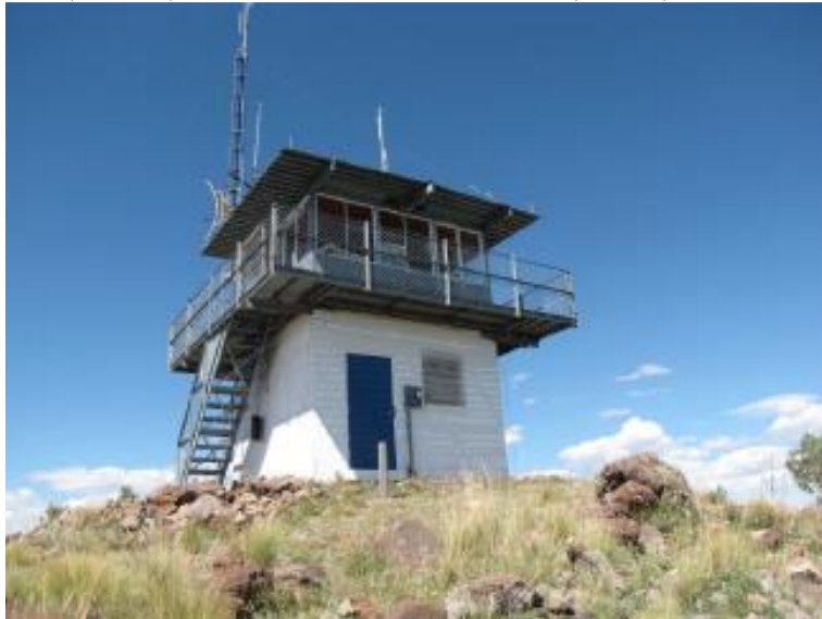
Current Cerro Pelado Lookout, an R6 flat CL-100. (2010, Courtesy of Janie O'Rourke)
