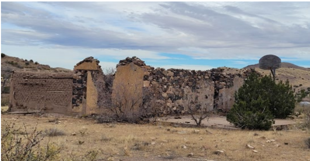
Old Nogal Ranch Building – Photo Credit: Jack Dickey
